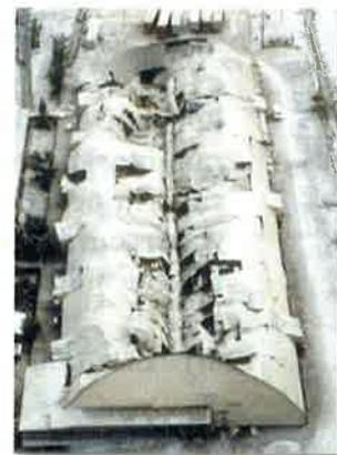
FIGURE 10 COLLAPSE OF A WAREHOUSE ROOF
