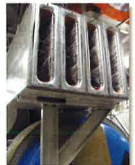
FIGURE 13 DIESEL GENERATOR INTAKE PRE-FILTER COWL
