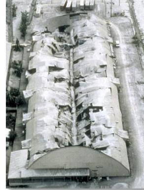
FIGURE 10 COLLAPSE OF A WAREHOUSE ROOF
