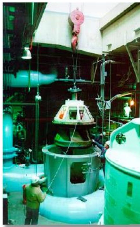
FIGURE 14 A MAIN CONDENSER COOLING PUMP, USUALLY ONE OF FOUR PUMPS
