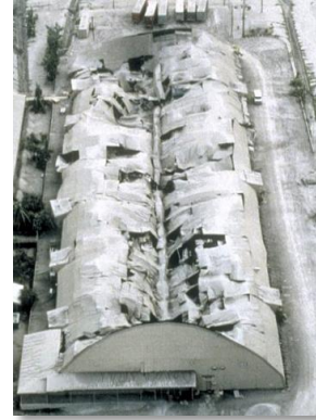
FIGURE 10 COLLAPSE OF A WAREHOUSE ROOF
