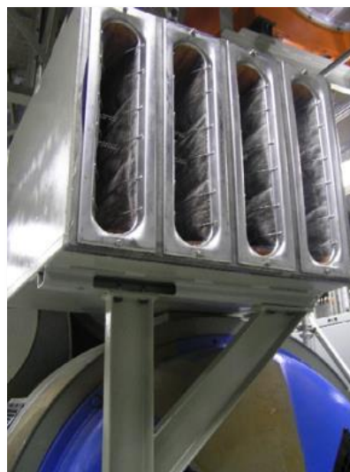
FIGURE 13 DIESEL GENERATOR INTAKE PRE-FILTER COWL
